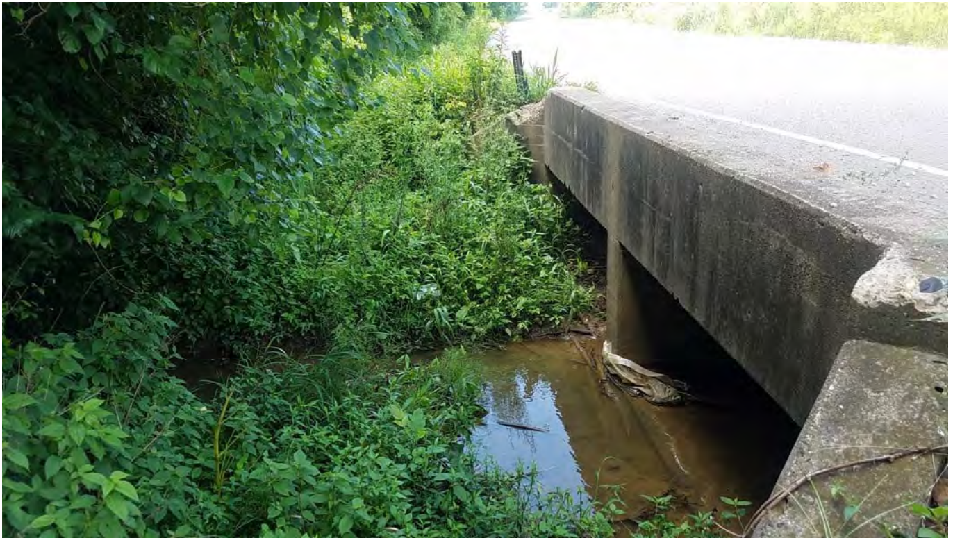
STR-27 Mound Slough (08/02/2017) Mound Slough passing through dual opening box culvert under Wolf Hills Road. Photo Direction: West
