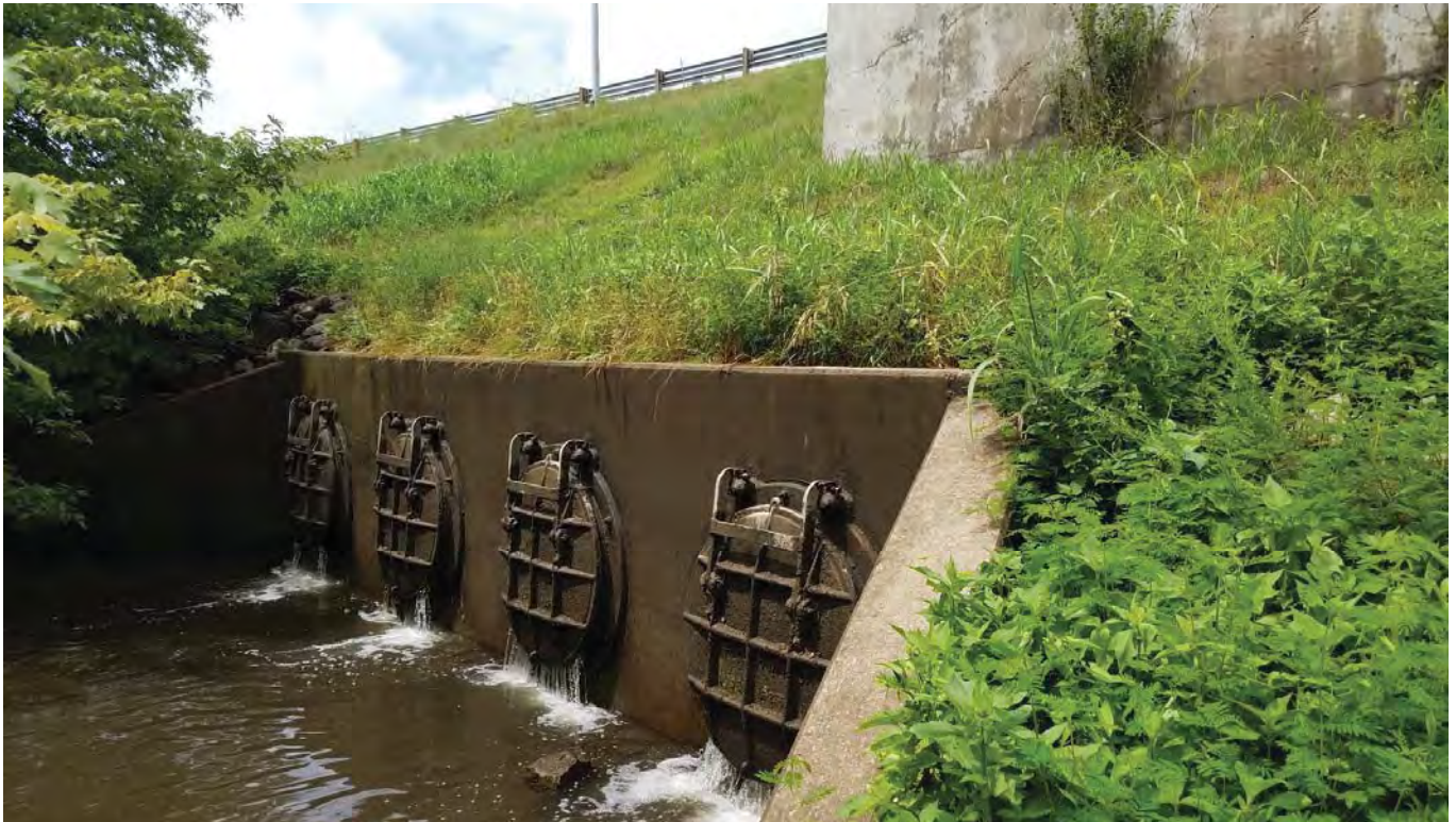
STR-12 Tributary to Eagle Creek (07/06/2017) Tributary to Eagle Creek showing the gated culverts under I-69. Photo direction: Northwest
