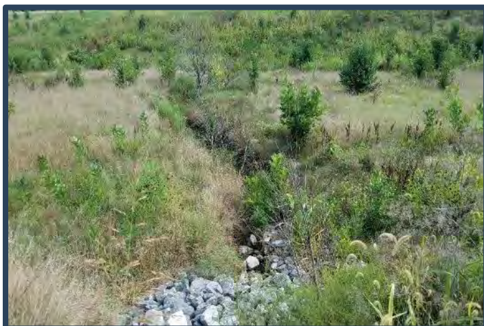
Photo 11: View of UNT-2 to Eagle Creek facing north. A portion of this channel is lined with riprap. The channel is deeply eroded/incised north of the riprap (08/17/18).
