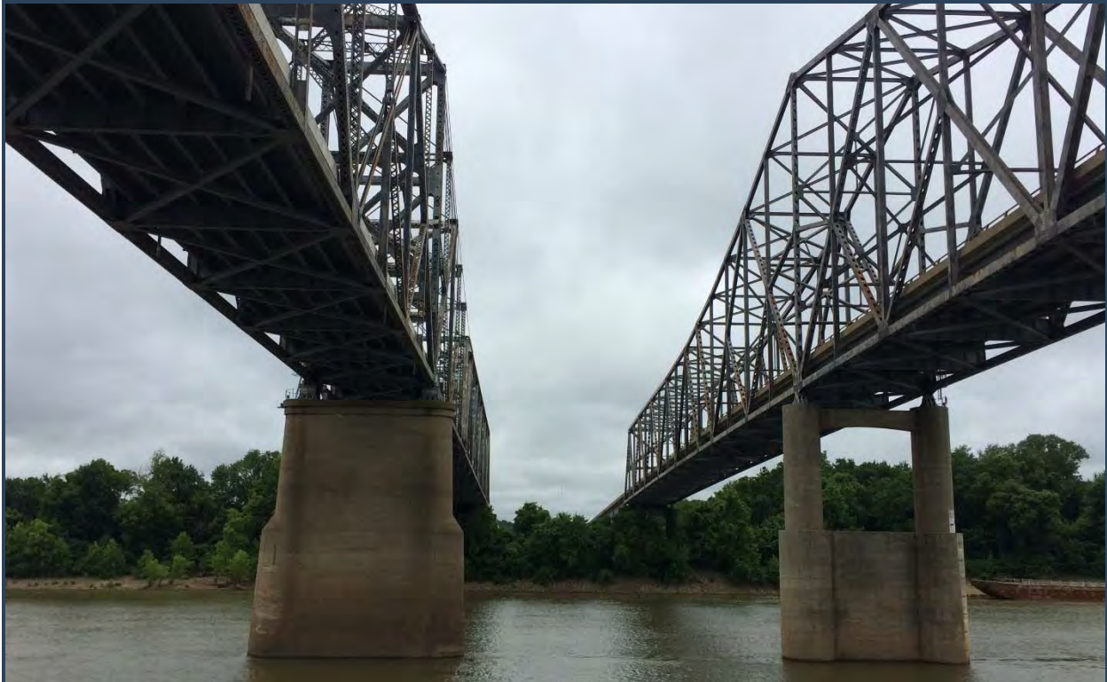
Figure 2. View South of the Through Truss River Span Units of the Ohio River Bridges (1932 Northbound Bridge at Left, 1965 Southbound Bridge at Right)
