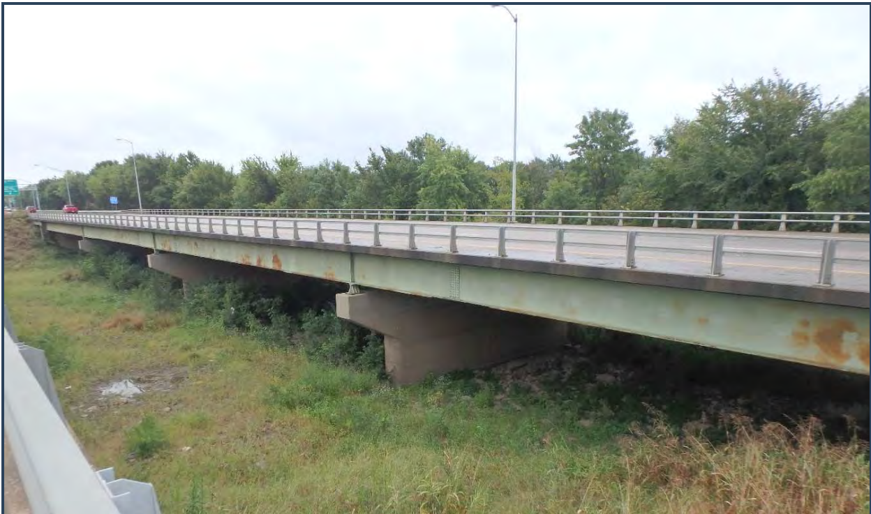
Figure 3. View North of Representative Overflow Bridge (NB 41 over Ohio River Overflow)
