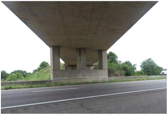
35. Looking west at intermediate pier of the substructure.
