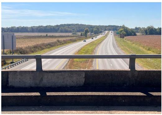
23. Looking south at bridge combination concrete parapet and metal piping railing and US 41 can be seen below.
