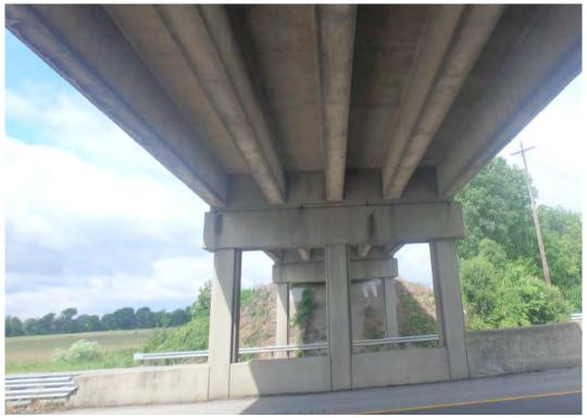
24. Looking at the one of the intermediate piers of the substructure supporting the tea beams and bridge deck above
