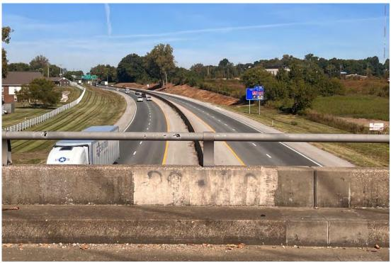
22. Looking north from the bridge at bridge combination concrete parapet and metal piping railing. US 41 can be seen below.
